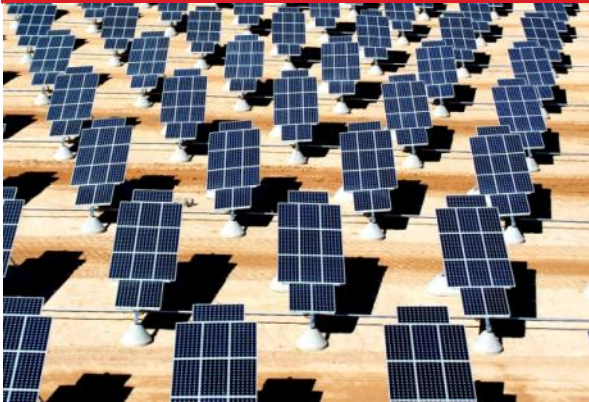
Photovoltaic Solar Power
