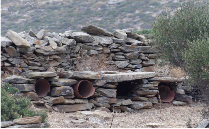
Fig. 11 Built-in hives of the modern era in a row in a dry stone wall, Kato Meri, Tinos island (photo by the author).
