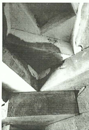
Fig. 6. Present-day view of the lantern roofing in the antechamber of the tomb at Strelcha (photograph N. Theodossiev)
